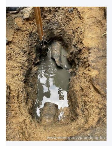
**4. Pipe Misalignment:** It can identify areas where pipes have shifted, become misaligned, or separated, which can cause issues with the flow of wastewater.
